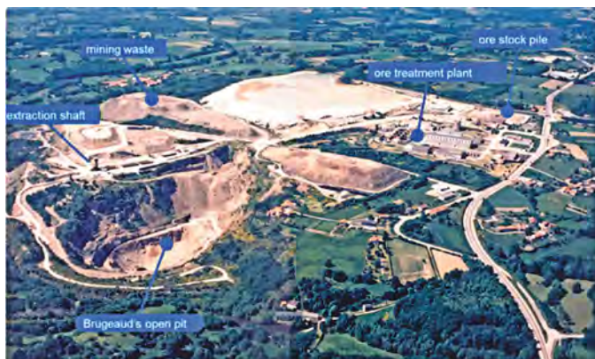
Fig. 3. Bessines uranium mine (France, 1978)
